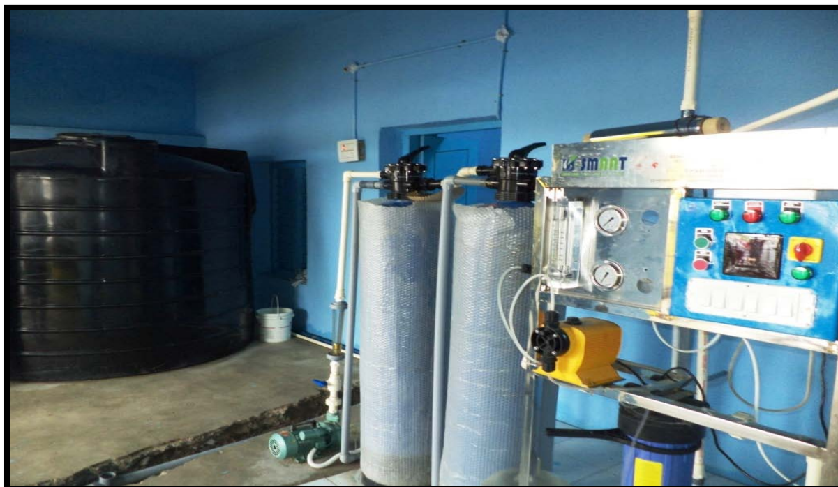
RO Water Plant provided in Srinagar village
